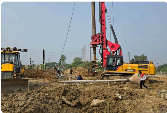
Piling at NH-76 ROB, Banda, Uttar Pradesh
