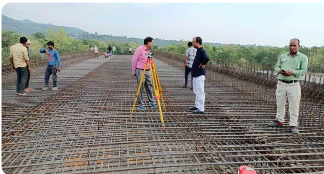
Engineers checking deck reinforcement with a total station
