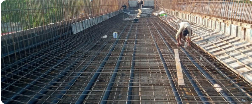
Pre-stressing ducts placed in deck reinforcement
