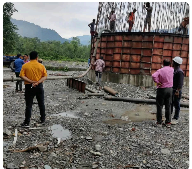
Well foundation steining in progress · Thano, Uttarakhand
