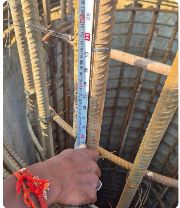
Checking pile cage reinforcement before lowering
