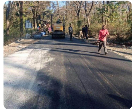
Bituminous road works
