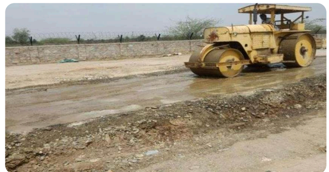
Earthwork compaction for road formation
