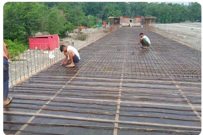
Deck slab reinforcement on a river bridge
