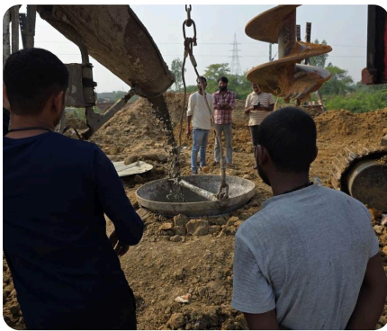
Pile concreting by tremie · NH-76 ROB
