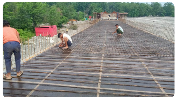
Deck reinforcement laid and tied for inspection
