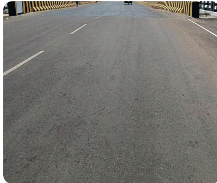
Completed deck · NH-930 bridge
