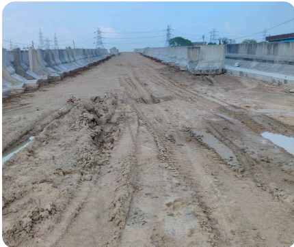
RE-wall approaches · NH-76 ROB
