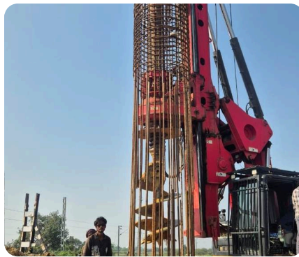
Lowering a pile reinforcement cage
